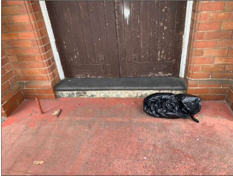
Figure 36: Coloured concrete floor of the porch and slate threshold to the door.
