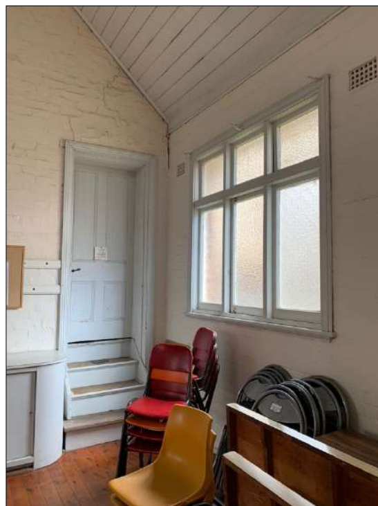
Figure 57: Window and door in the western wall. The door leaf has been replaced.
