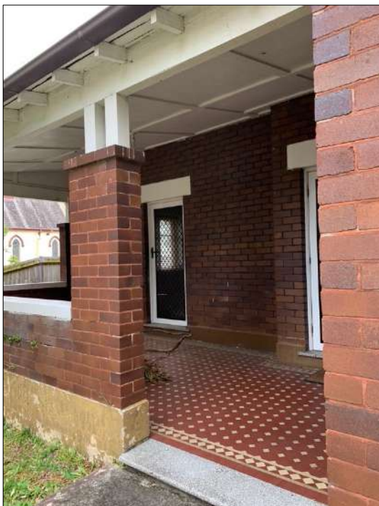
Figure 65: Detail of the front porch, showing the terrazzo threshold, enaustic tiling and battened f/c ceiling.
