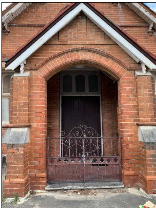
Figure 32: Northern elevation of the porch. Note the cement capping to the piers, the simple decorative brickwork to the gable and arch, the decorative brackets to the bargeboards and slate threshold into the porch.
