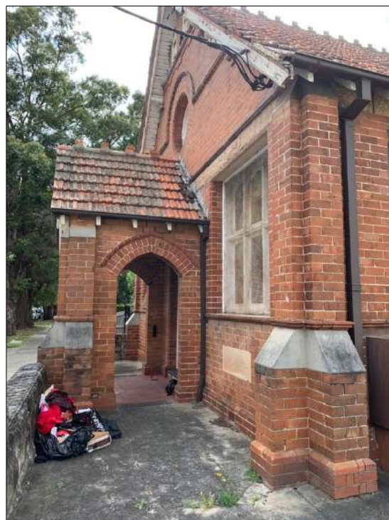
Figure 32: Northern elevation of the porch. Note the cement capping to the piers, the simple decorative brickwork to the gable and arch, the decorative brackets to the bargeboards and slate threshold into the porch.
