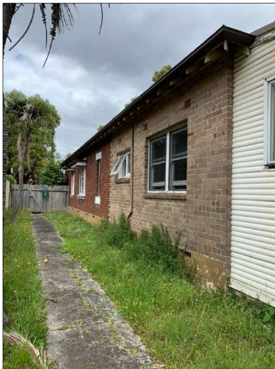
Figure 70: The southern elevation showing the transition between the dark brick and the common brick to the rear.
