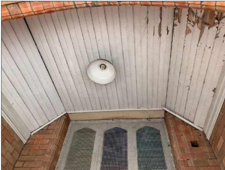
Figure 37: Timber lined ceiling.
