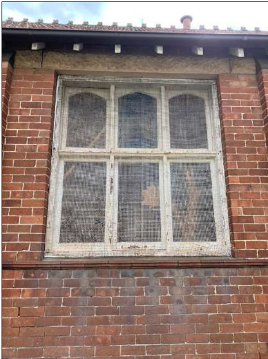
Figure 40: Detail of a window in one of the bays. Note the use of moulded brick below the opening.
